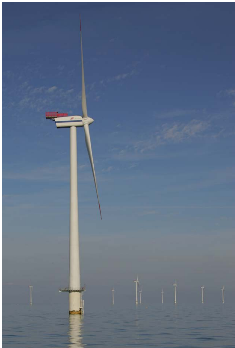
Horns Rev 1 Vestas turbine
